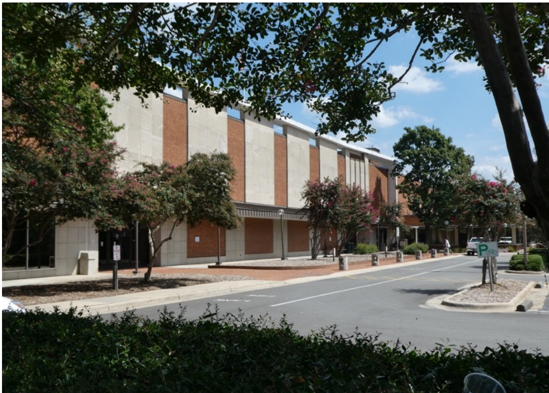
The Hal Marshall Center's main building – former Sears department store – in 2018.
